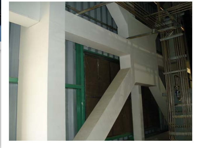
PROMATECT®-H structural steel column and beam cladding at the One Shelley Street office building (above) in Sydney, Australia and Tatan Power Point, Taiwan (left).
