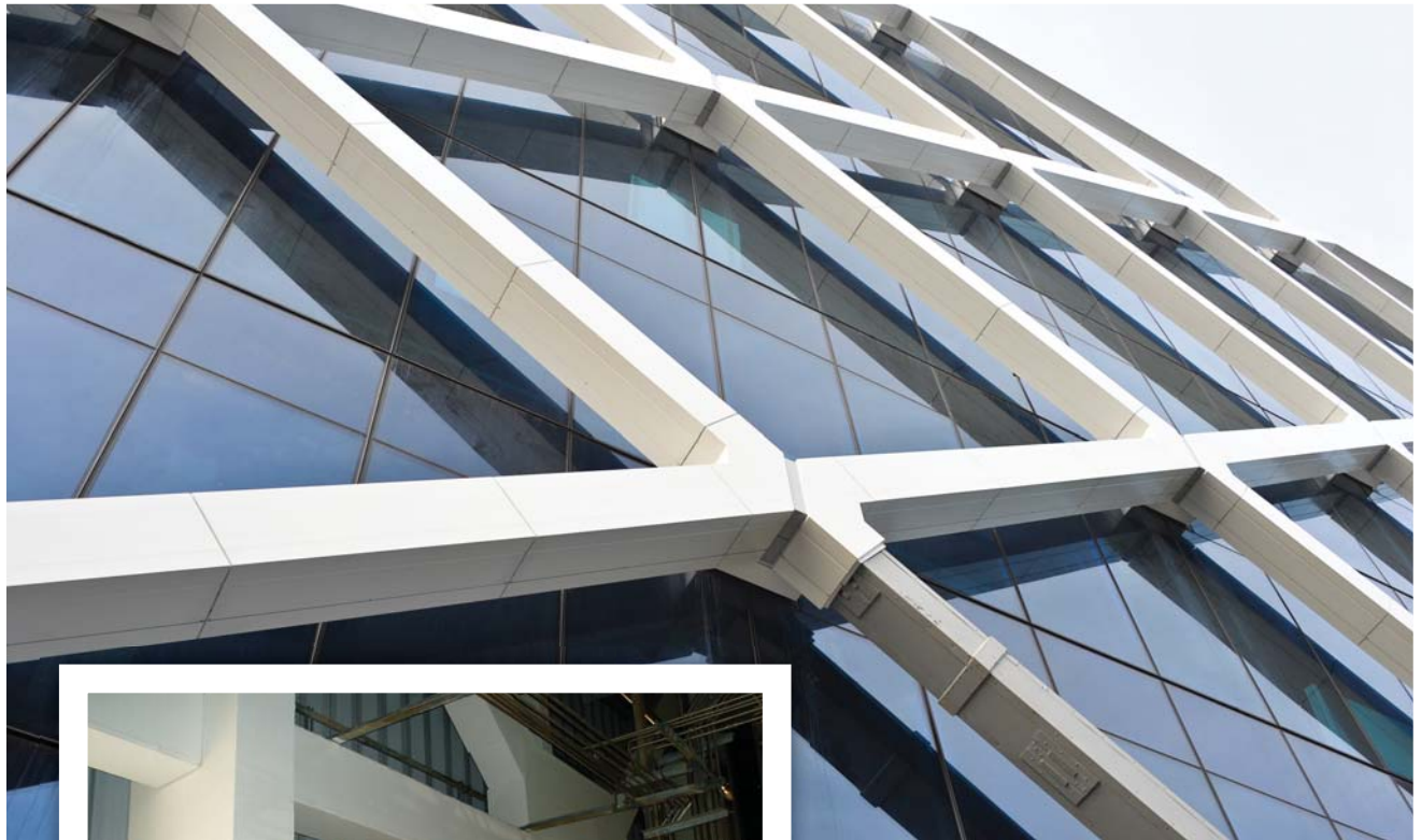
PROMATECT®-H structural steel column and beam cladding at the One Shelley Street office building (above) in Sydney, Australia and Tatan Power Point, Taiwan (left).
